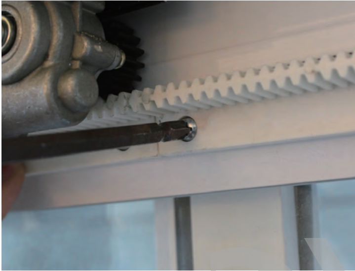
Installation of Mecahnism 2 (Top mounting)
