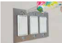
5. Adjust switches to level them out.
