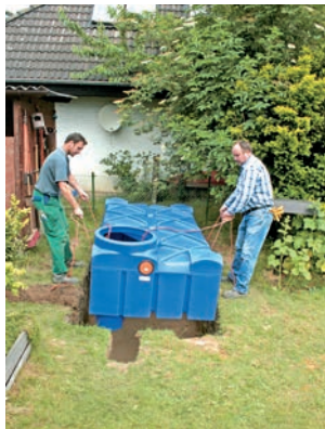
Place Lightweight tank is easily placed in the narrow and shallow pit.
