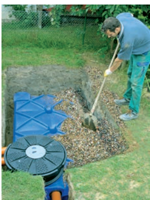
Backfill After assembling the components, simply backfill the pit, very little workspace required.
