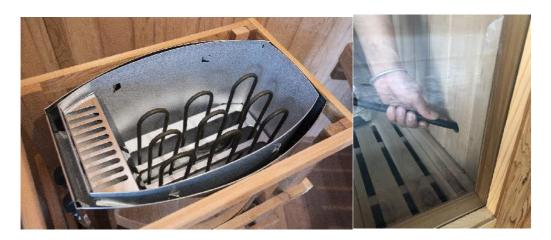
Insert the stove cable through sauna side wall hole.
