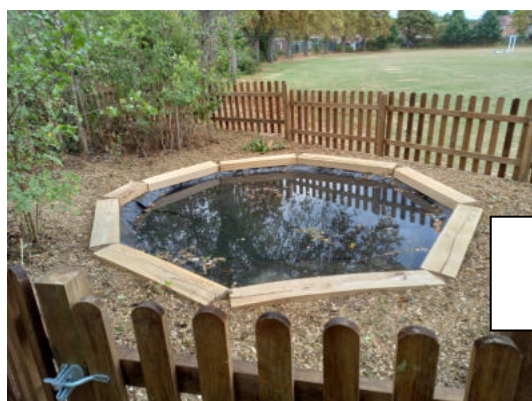
Ongoing work to the pond area.
