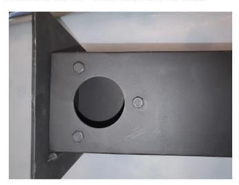
8.Attached the exit flue pipe using the 3 x screws. Do not tighten the screws until all 3 screws are in place.
