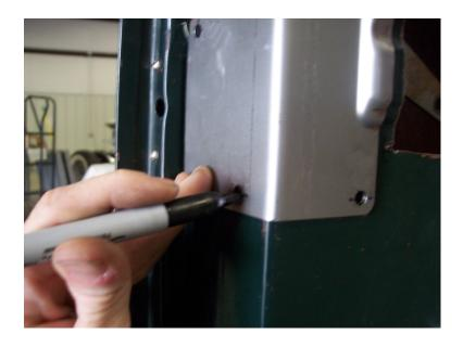
6. Mount the latch to the jam plate. Use 2 of the provided 1/4-20X1-1/4 stainless button head bolts in the upper latch mounting holes. These bolts will pass through the 2 slots on the latch slide plate. Use 2 of the provided 1/4-20 locking jam nuts to hold the plate flat to the latch. Do not overtighten the nuts. When actuating the latch using the outside handle, the slide plate should be free to slide, but not lift from the latch.
