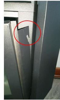
The glass panel is hooked by 2 hooks on each side.
