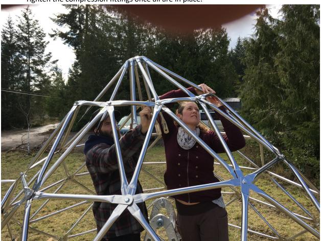
9. Temporarily tension the door frame together with some ratchet straps while going around and tightening all the nuts on the dome.
