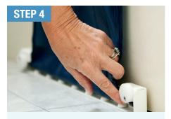
By rotating the discs the floor anchor rod can be located into the floor bracket itself. Turn the discs to ensure the floor anchor rod is positively locked in.
