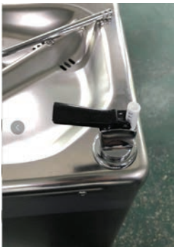
Glass filler installation
