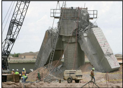
Demolition of Highway Bridge
