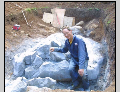
Swimming Pool Excavating
