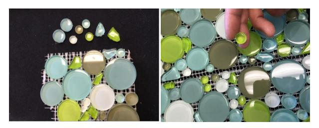
4. Fill the leftover gaps using the loose pieces; repeat process. Surplus of 10% is recommended.
