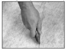
4.6 Chalk lines or other layout methods are easily applied over the light-coloured Mapeguard 2 surface.
