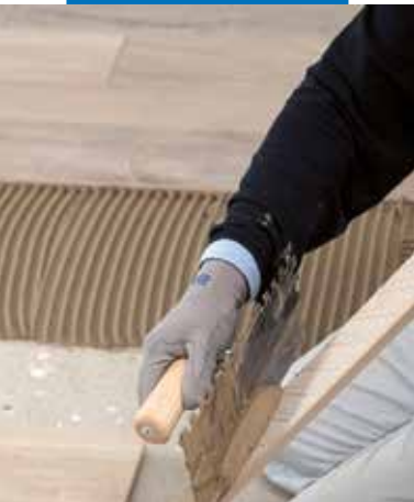
Application with the back-buttering technique
