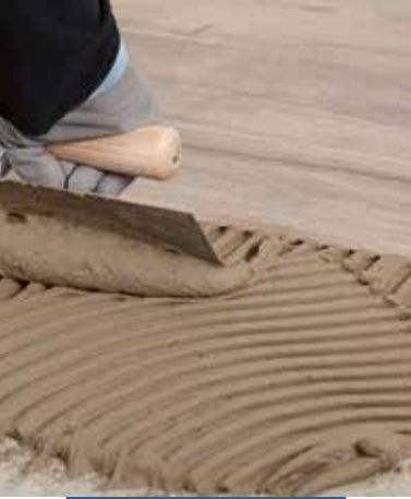
Bonding "imitation wood" effect porcelain floor tiles
