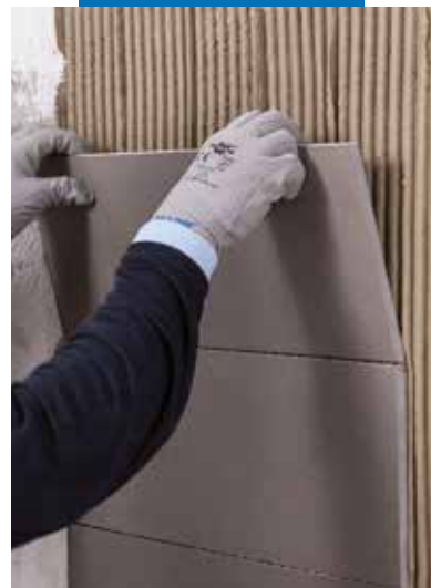
Installation of porcelain tiles on the wall
