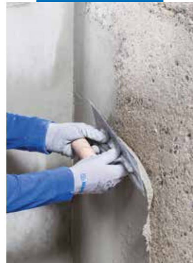
Applying Planitop Smooth & Repair R4 with a trowel
