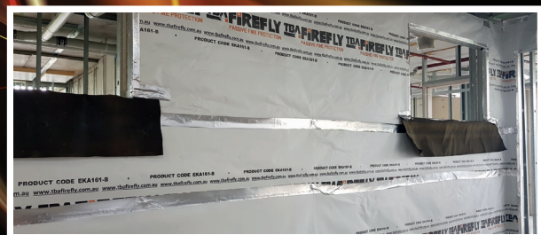
TBA Firefly™ Aluminium Foil Reinforced Tape Installed onto the Joints of the TBA Firefly™ Non-Combustible Sarking
