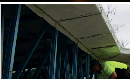
Sarking Under Eave Protection
