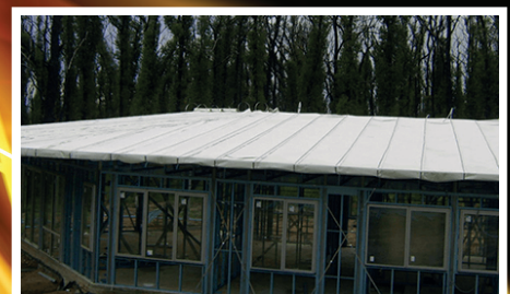
Completed Sarking Installation
