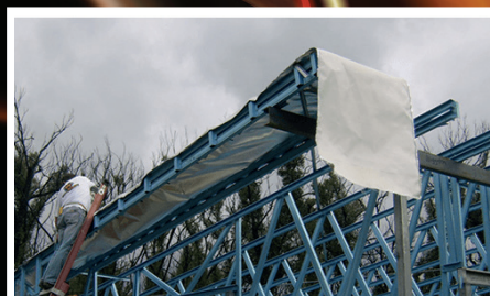
Starting Roof Wrap
