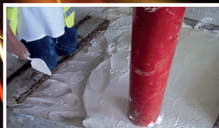
Trowelling up the Intucompound ® Seal
