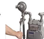
meter inlet valve, **do not** use pipe wrench.
