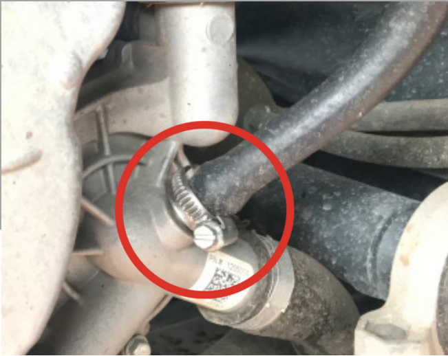
11. Install new coolant line from water pump to turbo
