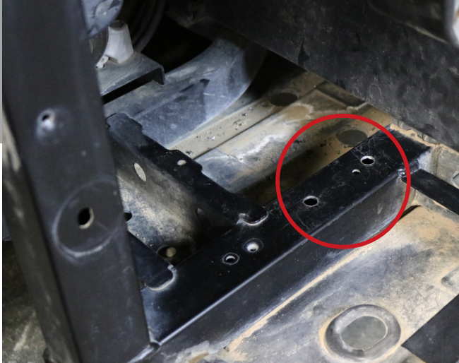
3. Under right hand quarter panel that was removed, drill two 3/8" holes for oil pump bracket
