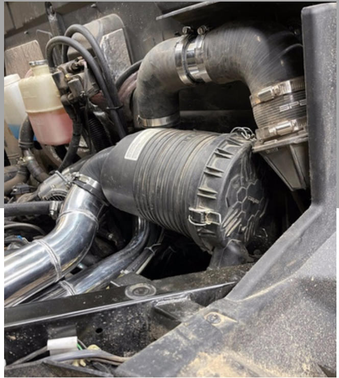
22. Install U bend silicone fitting assembly to top of the air filter box. Tighten down clamp
