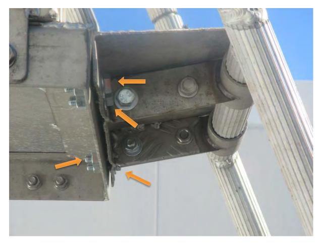
Step 3: Unbolt and remove platform-ladder connection
