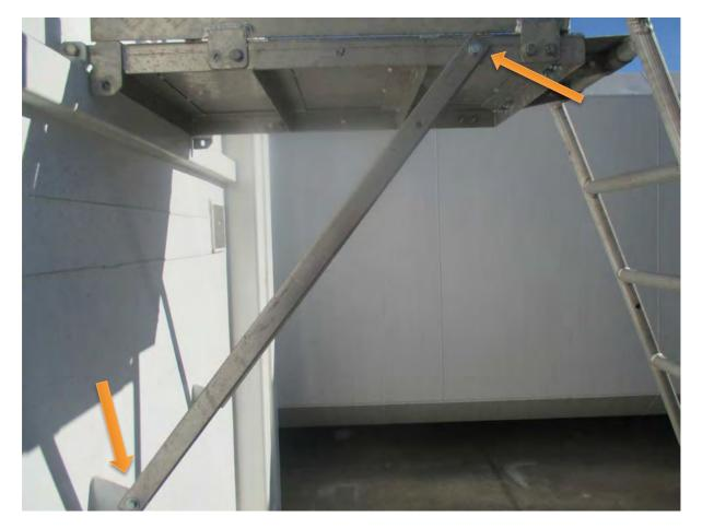
Step 2: Unbolt and remove supports from platform and tank brackets
