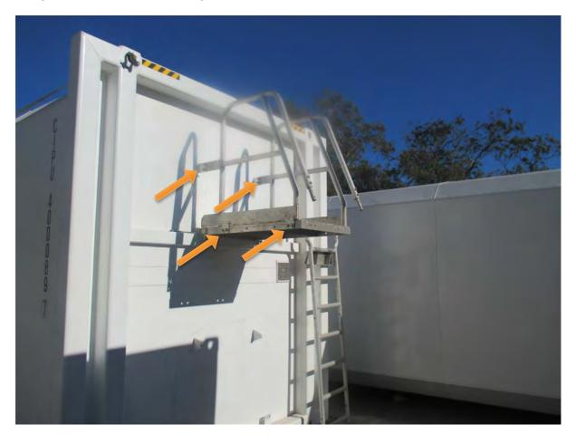
Step 2: Bolt handrails to platform and tank brackets.
