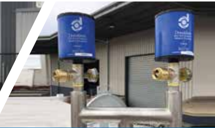
Tank Air Breather Filtration
