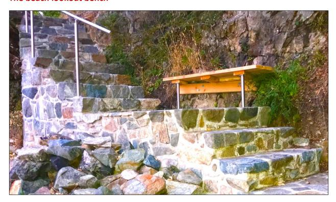
For the lookout bench on the main landing, just above the beach at the bottom of the long set of railed steps, the bench lumber is durable native Western Red Cedar. Especially since the cedar may need replacing every few decades, the whole bench structure is designed for efficient removal—as a single unit—for restoration when that is eventually needed.
