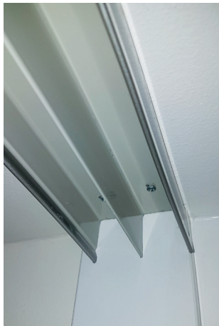
Strike plate or end panel, showing top track & fixing block to ceiling
