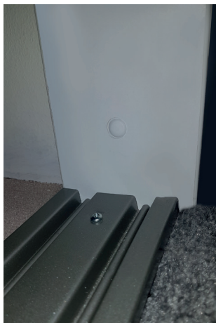
Skirting board cut out for strike plate
