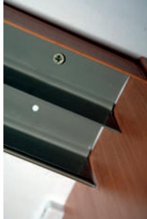
top track butting up to end panel showing ceiling fixing
