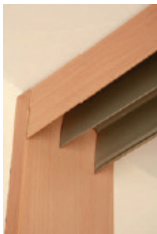
Top track butting up against a strike plate
