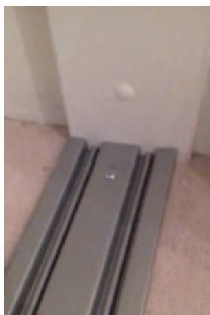
Skirting board cut and strike plate attached to wall
