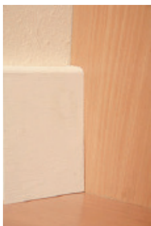
Skirting board fit up to end panel
