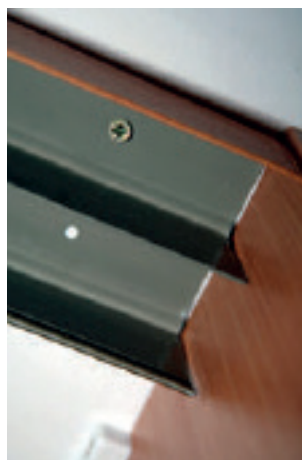
top track butting up to end panel showing ceiling fixing top track butting up to end panel showing ceiling fixing
