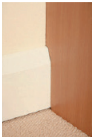
End panel scribed around skirting board
