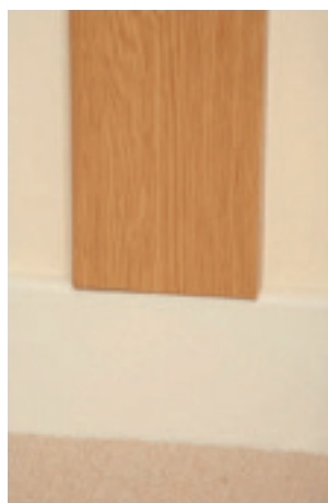
Strike plate fitted above skirting board
