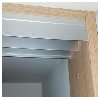
Strike plate or end panel, showing top track & fixing block to ceiling
