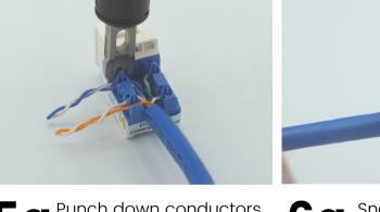
**50** Punch down conductors using trueIMPACT tool.
