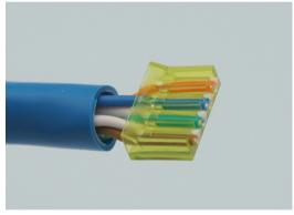
Load bar installed properly and conductors flush cut, T568B sequence shown.
