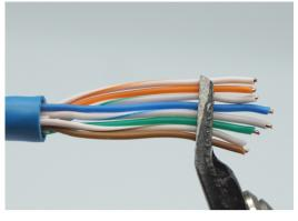
Remove kinks and place conductors into order, T568B shown. Flush cut.
