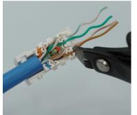
Carefully flush cut conductors even with conductor holder cap as shown. Cut conductors vertically, one at a time. Do not accidentally cut off the white locking tabs!
