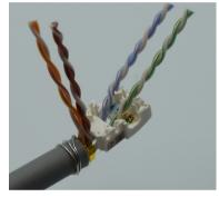
5 Slide wiring cap towards cable jacket. 2 conductor pairs go below bar and 2 above according to color code.
