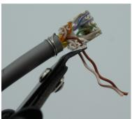
**7** Flush cut off conductors even with the cap housing.
