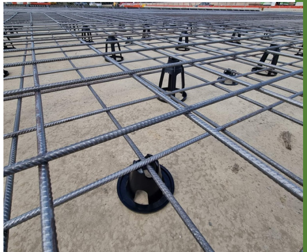
Figure 08 Bar chairs supporting reinforcement.
