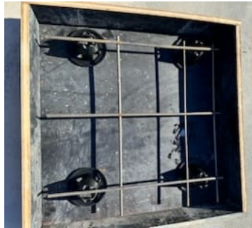
Figure 07 Bar chairs supporting reinforcement during concrete
