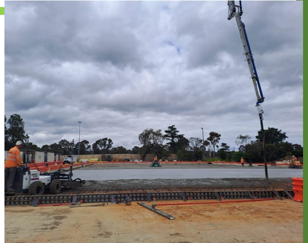
Figure 07 Bar chairs supporting reinforcement during concrete
