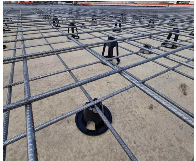
Figure 08 Bar chairs supporting reinforcement.
