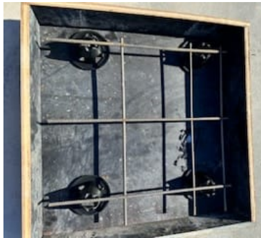
Figure 07 Bar chairs supporting reinforcement during concrete
