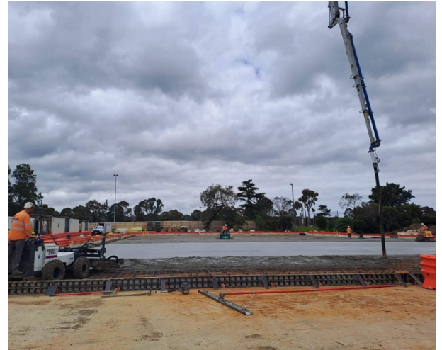
Figure 07 Bar chairs supporting reinforcement during concrete
