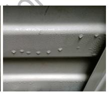
The most basic rule that never changes is this: **moisture (also called condensation) occurs when relatively warm-moist air comes in contact with a relatively cold surface.** The key word here is "relatively" because condensation can occur at pretty much any temperature if given the right circumstances. However, for most metal buildings we are usually talking about when it's cold outside.
