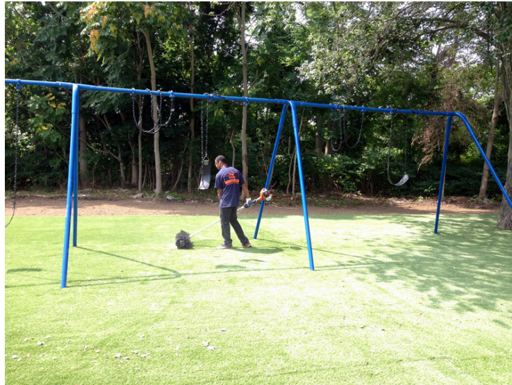
Spreading synthetic turf infill
