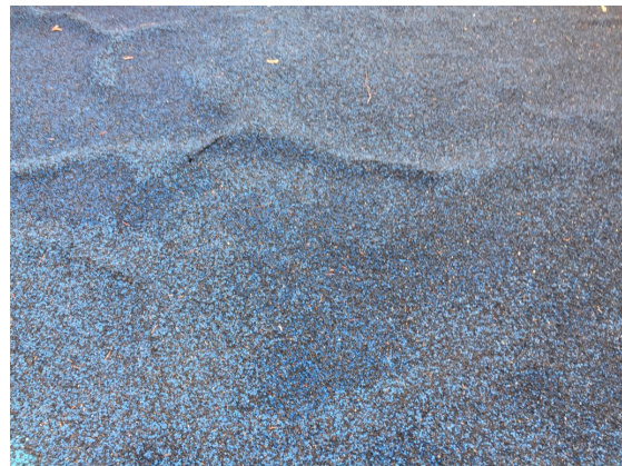
Wear layer ripple due to lack of proper bond with base layer
