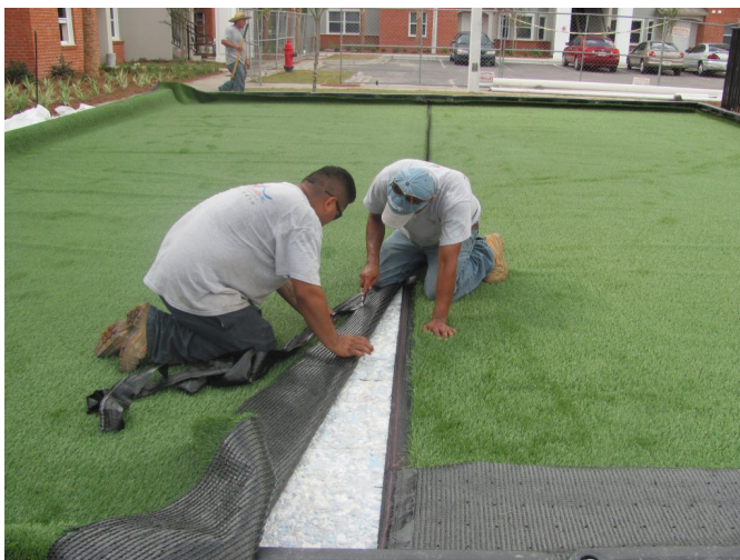
Seaming synthetic turf
