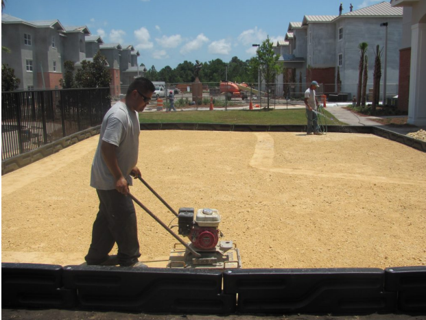
Aggregate compaction prior to installing the safety surface
