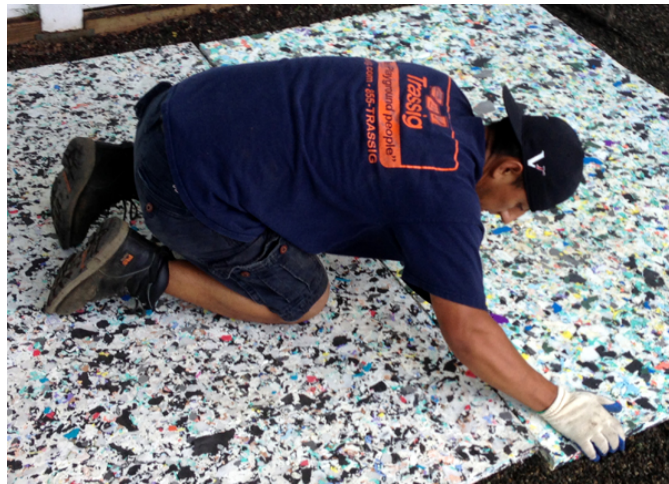
Installing synthetic turf padding
