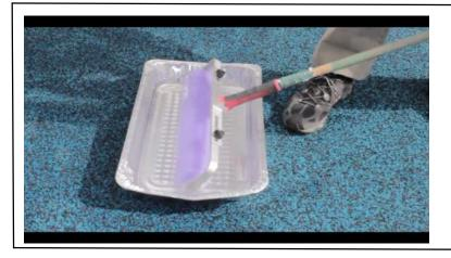
Step 4: Use a cheap paint roller to equally distribute Rebinder™ on your poured in place surface because you will be throwing it away after installation.
