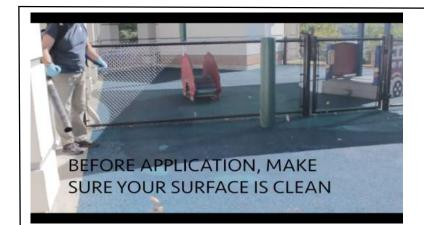
Step 1: Use a leaf blower to remove loose granulated rubber and other debris from area. If necessary, use a power washer with a wide angle nozzle and binder friendly detergent to sanitize the surface. Make sure your surface is COMPLETELY dry before continuing. Check under equipment for possible excess water and moisture
