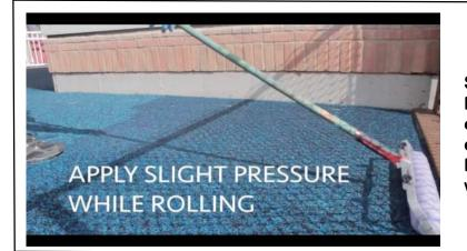
Step 5: Apply pressure when applying Rebinder™ in order to make sure the coat is even and sufficient. Go over each area only one time. Do not treat Rebinder™ like paint. Multiple layers will harden your surface.
