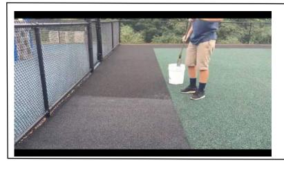
Step 6: Even though Trassig's Rebinder™ is fast curing, secure area and allow 24 hours before use after application. If it rains 4 hours or more after application the Rebinder™ will not be affected, but it cannot rain during the application of the Rebinder™ for it to properly cure.
