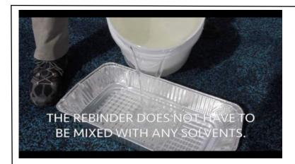
Step 3: Pour Rebinder™ into drip pan. Do not mix with other products or solvents.
