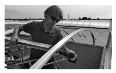
Fix without gaps between the crossbeams and LP525.
