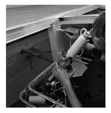
Push the power cable on the other side in the tube and make the electronic connection inside the tube in a junction box (not delivered) or use another connection method.
