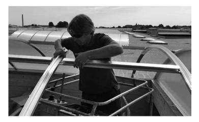
Fix the 4 crossbeams with 4 M6 x 70 mm bolts.
