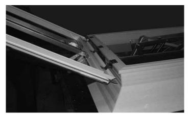
Close the dome and fix the hinge axes (1 per hinge).
