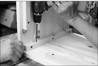
◄ Align the corners and attach the End and Side with glue and screws. Corner ribs should be flush with the top edge of the casket box.
