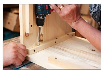
remaining long Side panel on the work surface. Position the other three sides on top of the remaining long Side panel and attach with glue and screws. Align the sides for a nice flush outside corner.
