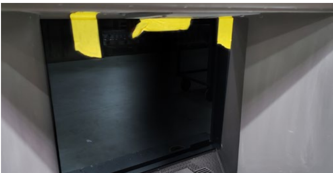
Figure 20.b hold it in place using masking tape
