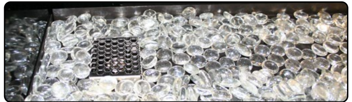
Figure 24.b Completed firestone installation
