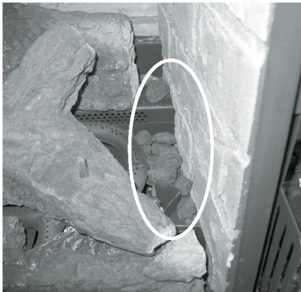
Right side of Burner
