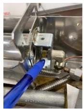
Once the orifice is installed, reinstall the air shutter in it's original location. Now reassemble the pilot assembly, the burner cover and pilot assembly cover. Slide the burner back in and put the front screw in and rear access panel. Be careful not to pinch the white igniter wire while putting the burner back in.
