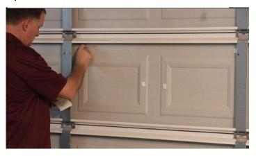
For improved thermal performance, add 3/4" air space between Reflective Air and door. This can be done by attaching to door framing rather than to the door panel
