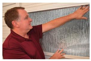
**Practice/Step 1:** It is best to use the extra size of the panel to help hold the panel in place. Simply "push" and "move" the panel in the proper position within the panel to the desired fit *(before using the Stick'ems™ adhesive squares!)* Once you "see" how the panels will fit proceed to the next step.
