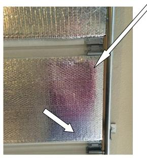
NOTE: There are eight (8) radiant barrier panels in the kit. Each panel is 4 feet in length. It is recommended that you use (5-6) Stick'ems<sup>™</sup> per panel. 48 squares are included in your kit to complete the installation.
