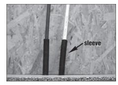
Protect pipe with non-metallic sleeves where it penetrates a slab or foundation.
