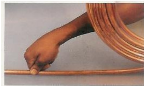
Figure 5-4 Tubing should be unrolled carefully to avoid kinking the pipe. Photo by Bill Johnson.
