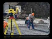
Layout points on blinding layer such as pipe insert or cut-outs before pouring concrete
